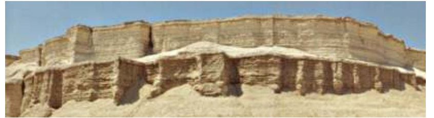
CITY WALLS - Eroded but discernible, the boundaries of the city are still there
